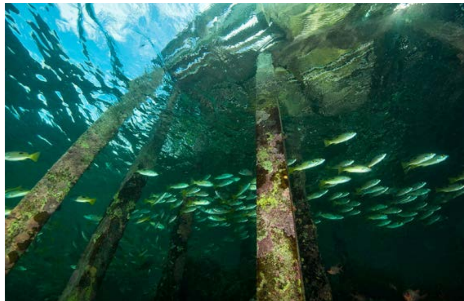
Underneath Uepi's Welcome Jetty; Reef sharks patrol at Uepi's Welcome Jetty (top right)
